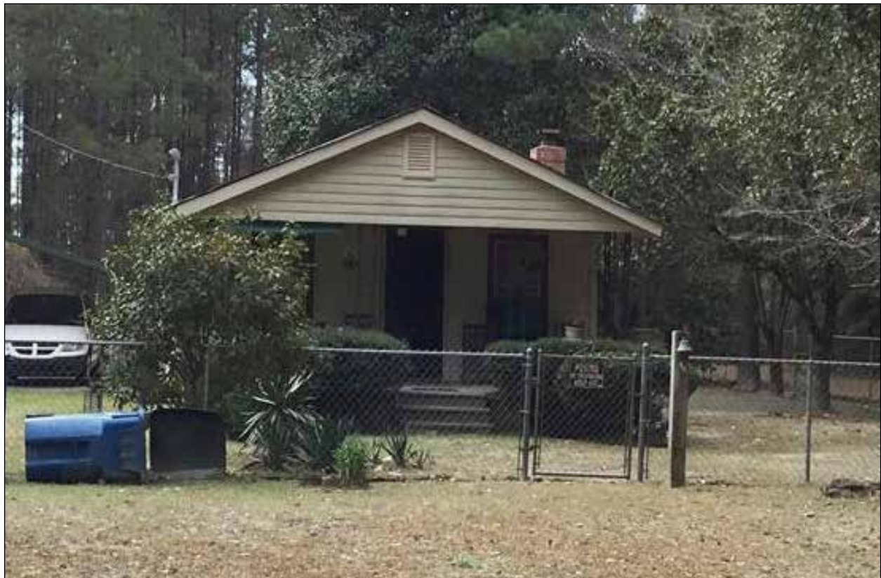
Figure 5.28 Resource 22, northeast oblique (Bryan County Tax Assessor 2017).
