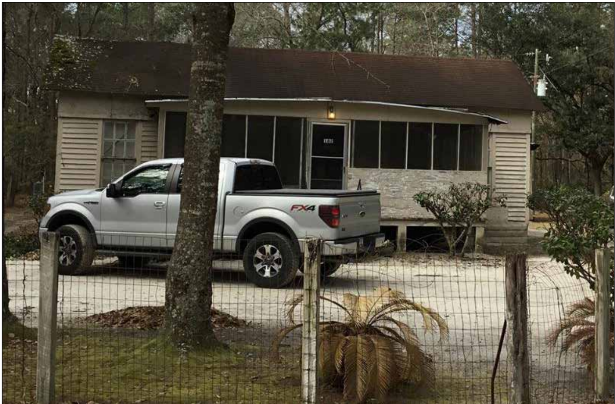
Figure 5.12 Resource 6, east (front) elevation (Bryan County Tax Assessor 2017).
