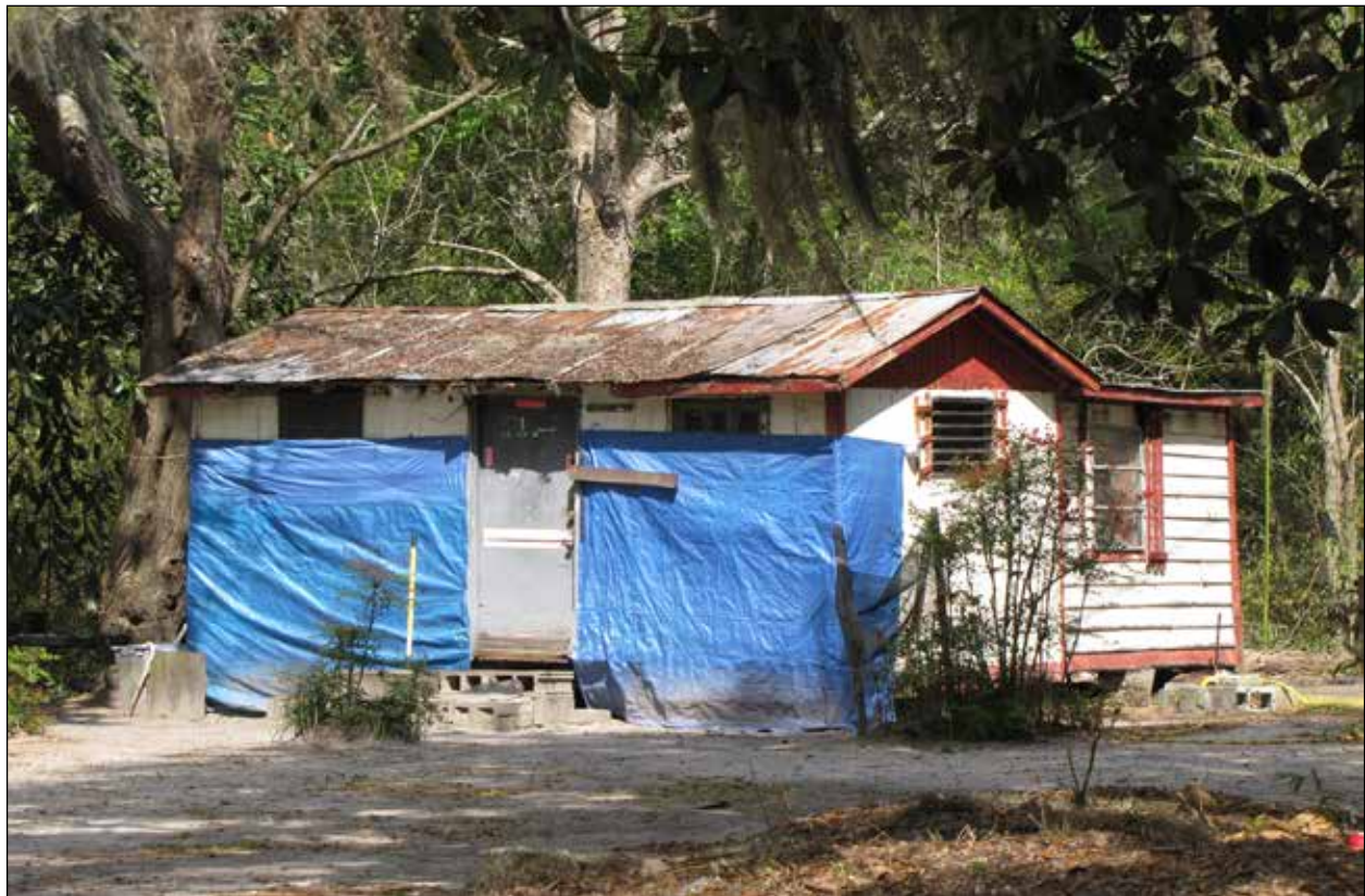
Figure 5.21 Resource 14, southwest oblique.
