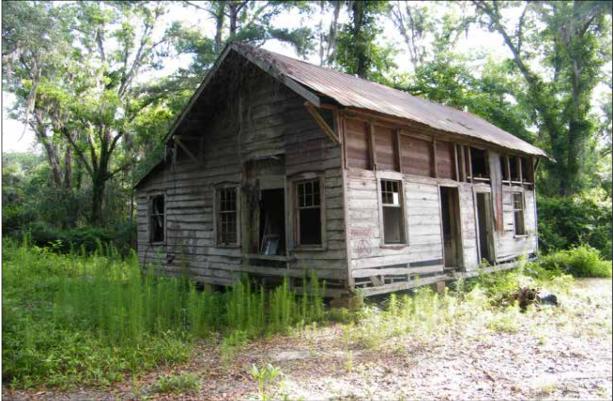
Figure 5.41 Resource 26.2, southwest oblique.
