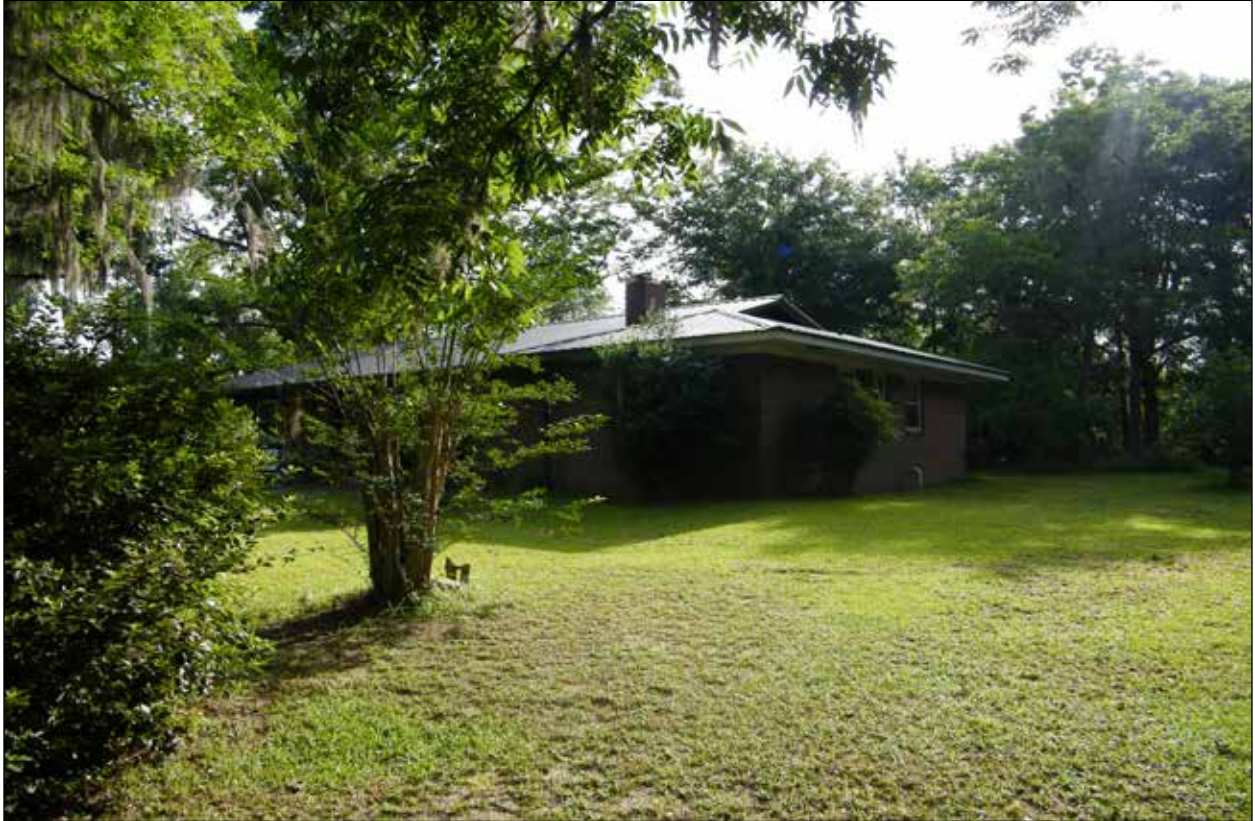
Figure 5.35 Resource 26, southwest oblique.
