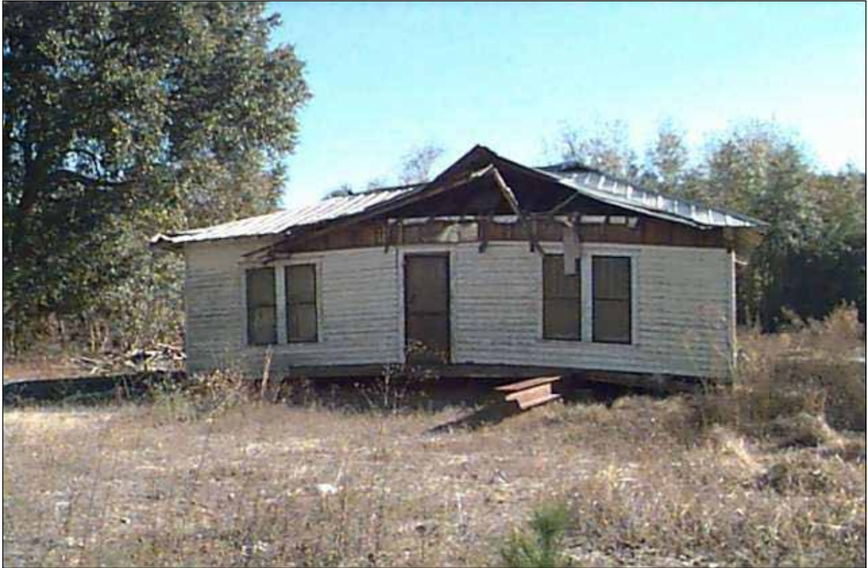
Figure 5.19 Resource 13, courtesy of Bryan County Georgia Board of Assessors.
