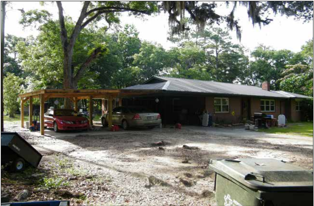
Figure 5.36 Resource 26, carport extension, northwest oblique.
