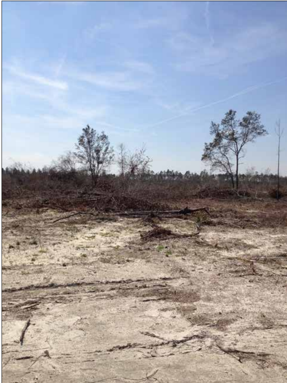
Figure 2.10 View of recently cleared areas, looking northeast toward I-16; pedestalled hardwoods give an indication of the extent of soil disturbance.
